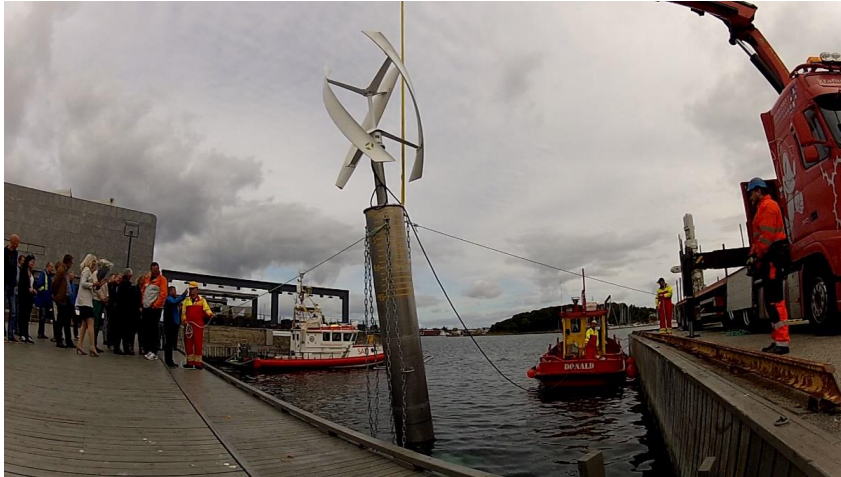
Figure 1. Gwind floating VAWT pilot project in Stavanger. Photo: Simen Malmin
